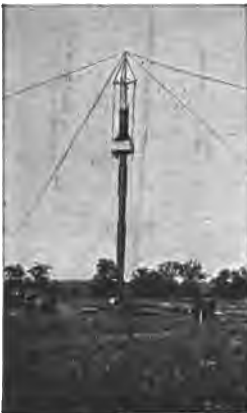
Fig. 313—A Tubular Mast in Early Stages of Construction.
